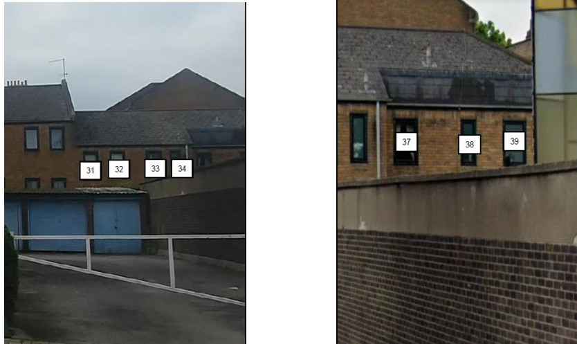
Figure 14 – Windows tested at 10-17 Searle Place
