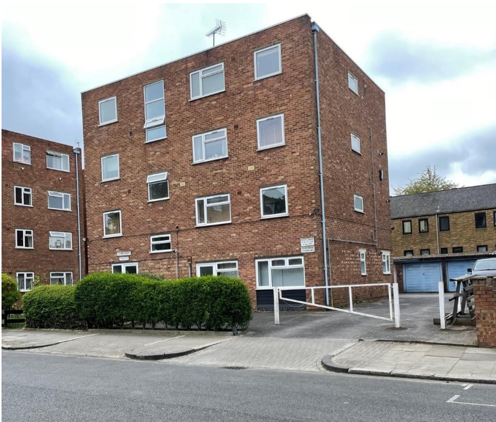
Figure 4 – Street View from Regina Road
